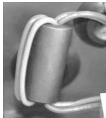
Figure 3-2: Ferrite core and battery supply wiring
